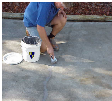
Picture: Slab Repair applied by Spatula. Slab Repair comes in various sized pails.
