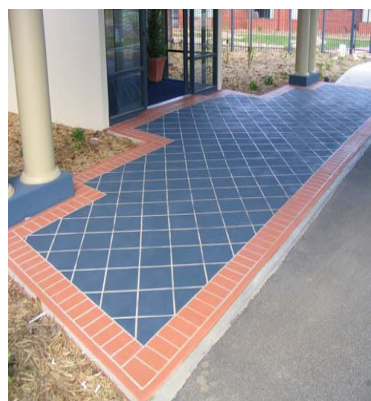
Top Picture: Covercoat W applied to Stencilshield with airless spray and 517 tip.
